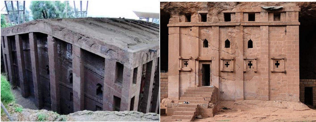
Figure 12: Level of Damage in Bete Medhane Alem (House of the Savior of the World) & Biete Abba Libanos (House of Abbot Libanos)
