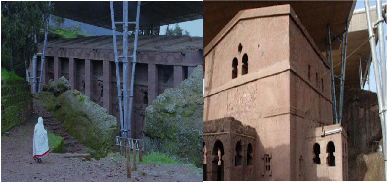
Figure 8: European Union’s Shelters Installed to Protect from Water Infiltration
