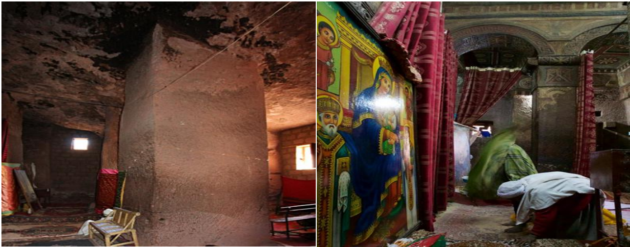
Figure 2: Original Features are Severely Damaged and Hardly Recognizable in Biete Mariam (House of Mary) Church
