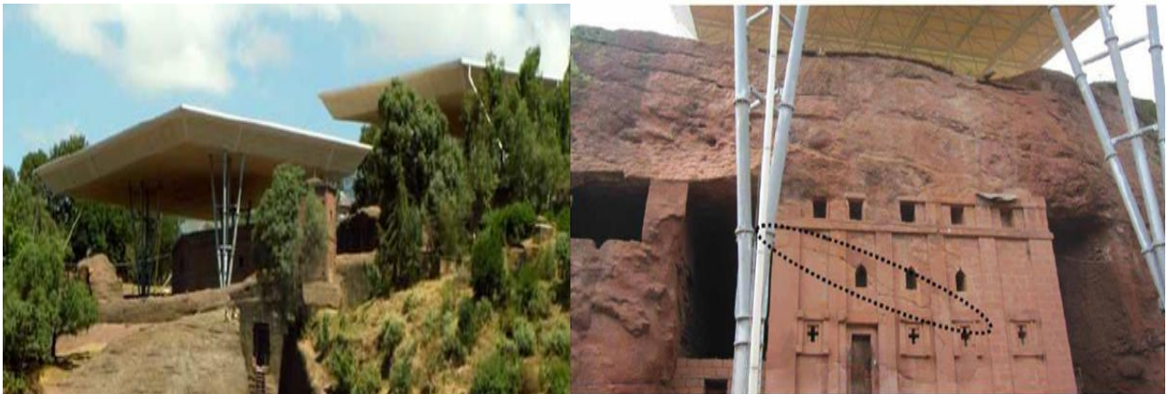
Figure 6: Temporary Shelters Installed to Protect Five Churches from Water Infiltration
