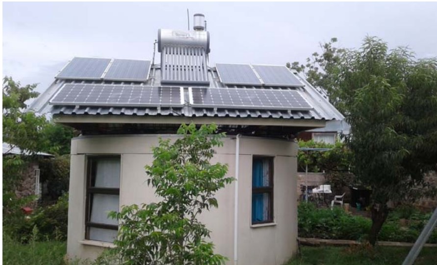
Figure 23. Rotating roof for augmented power and hot water supply adjacent to the bakery. Roof orientation depicted is straight east and provides good power soon after sun-rise for operating the dough mixer.
