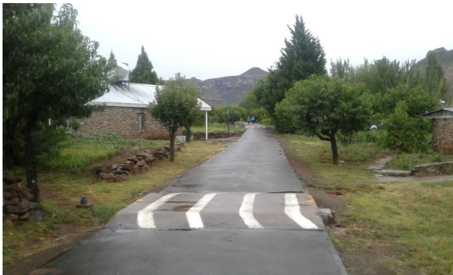
Figure 11. Paved lane through the BBCDC campus with four speed bumps/water management features.
